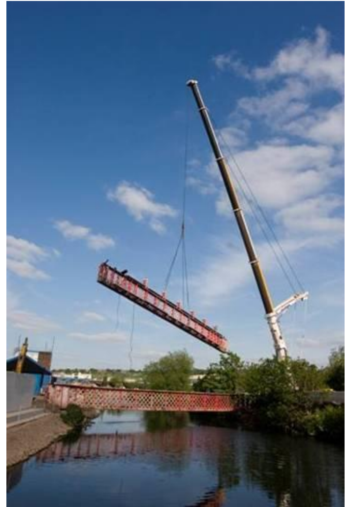
Removal of redundant bridges
