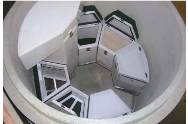
Exhibit 2.35 Proprietary Up-Flo filter system from Hydro International
