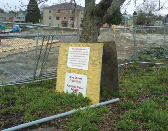
Exhibit 2.33 Protecting established trees
