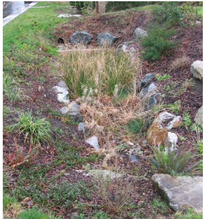
Exhibit 2.25 A typical bio-swale located in a residential garden
