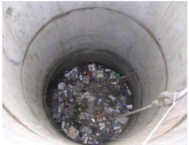
Exhibit 2.41 The captured contents of a CDS separator prior to annual clean-out
