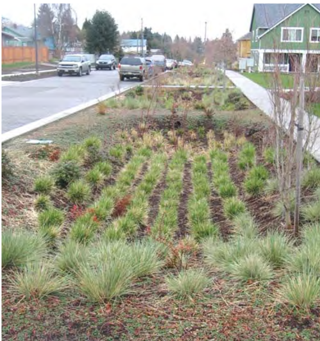
Exhibit 2.22 A SEA street bio-swale edged with porous road and pavement
