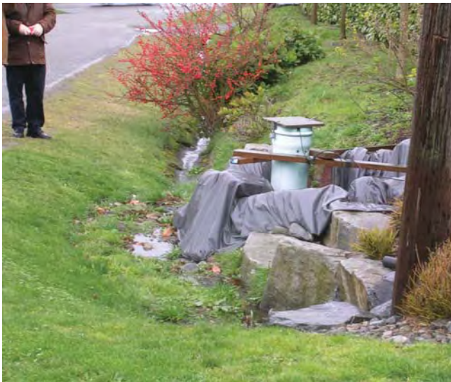
Exhibit 2.40 Temporary monitoring equipment in place at SEA Street development
