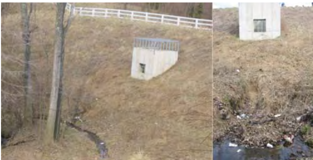
Exhibit 2.5 Example of poor maintenance
