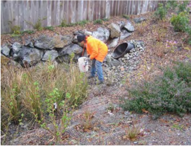
Exhibit 2.3 Maintenance and cleaning
