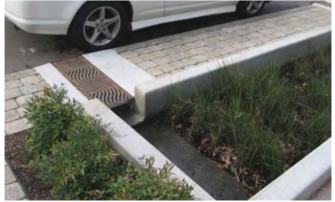
Exhibit 2.21 An inlet to the street planter and note integration with pavement
