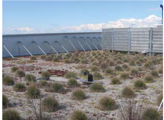
Exhibit 2.16 An impressively vegetated green street eco-roof
