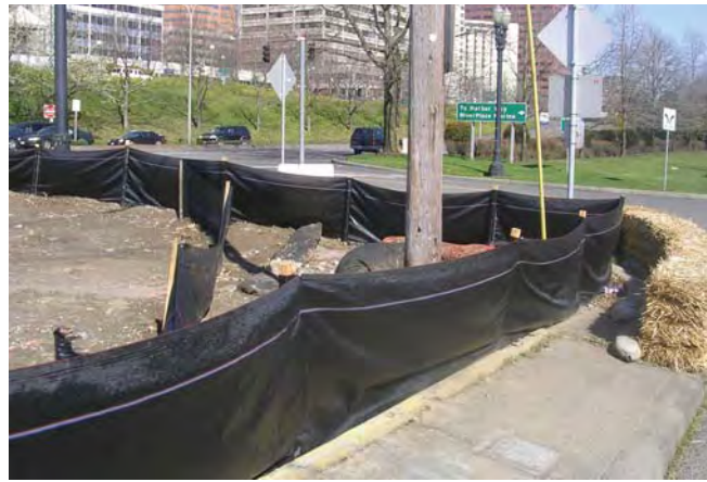
Exhibit 2.36 Sediment control on a construction site in Portland, Oregon
