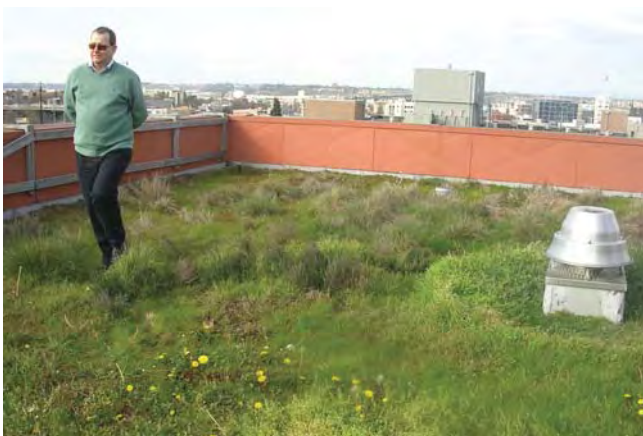
Exhibit 2.34 Green-roof in Portland, Oregon
