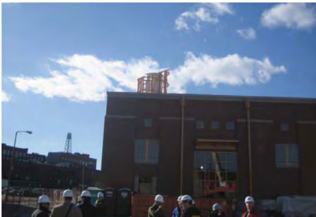
Exhibit C.10 Union Park Detention Treatment Facility
