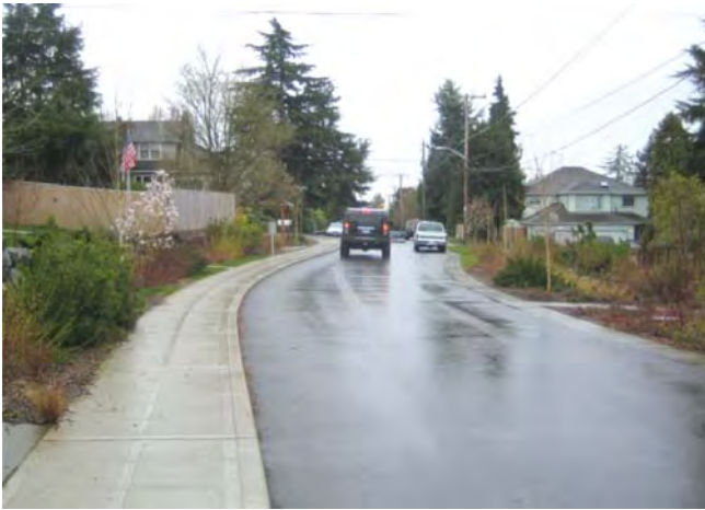
Exhibit C.16 Post construction of SEA street
