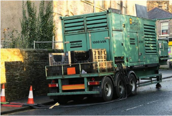
Figure 5: Generator in Lancaster, connected to local substation
