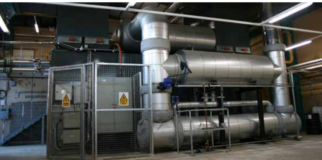
The CHP in the Energy Centre
