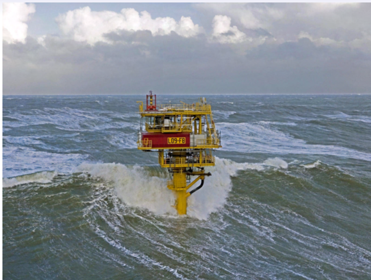
"L9" platform in the Southern North Sea.
