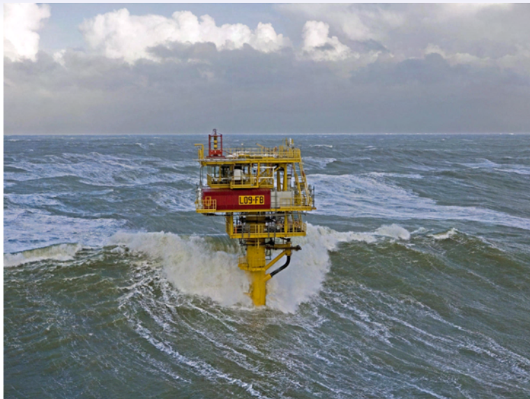
"L9" platform in the Southern North Sea.
