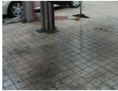
Figure 15: Build up of dirt in a highly controlled environment
